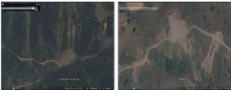
Figure 4: Damage to road from earthquake due to triggering of old landslide as well as development of new landslide in Dhading (left image before earthquake and right image after earthquake)
